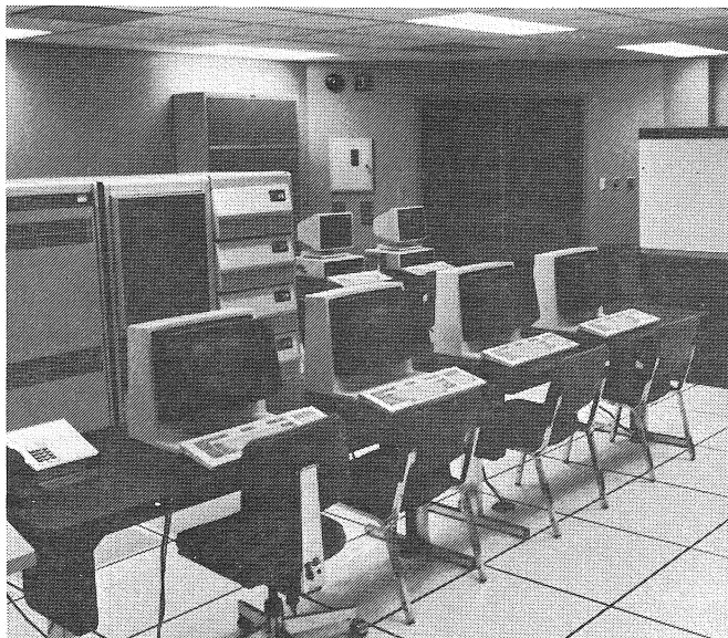
Machine room, Nichols Hall
