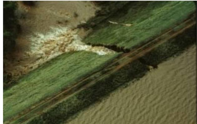
**Figure 1.** Internal erosion of USDA-NRCS structure
